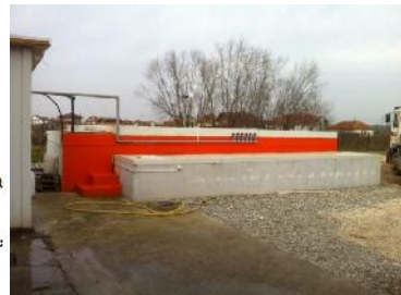
Fig. 1.1. Sequencing batch reactor in dairy industry (Vingneswaran et al., 2007).
